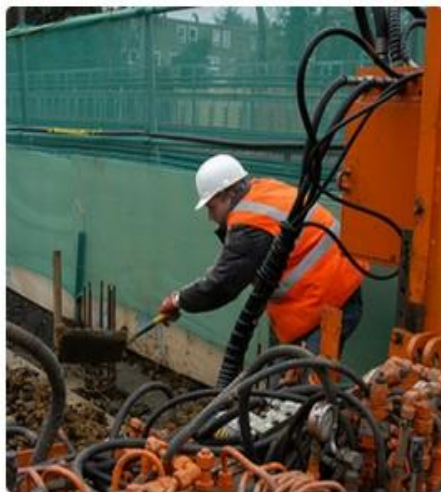
"construction worker in orange safety vest is working on road."
