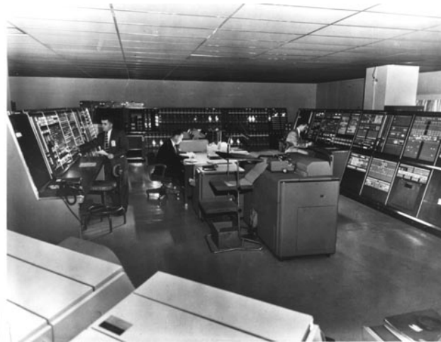
SAGE Control Room
