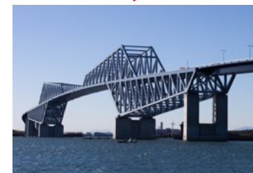
Tokyo Gate Bridge
