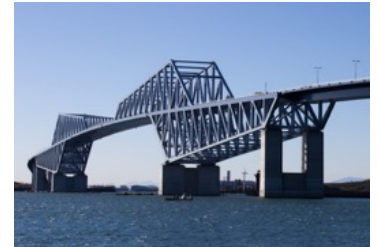
Tokyo Gate Bridge
